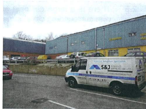
Rear of Site Looking West
