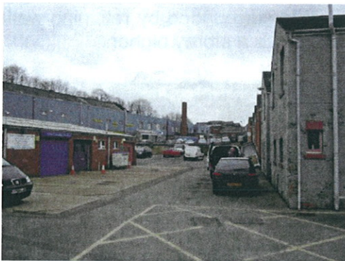
Rear of Site looking North
