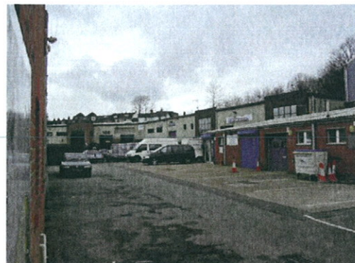
Site looking South to Vehicular Entrance new Industrial Unit West
